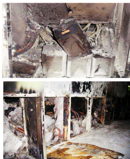
Figure 1: Damage to the voltage transformer.
